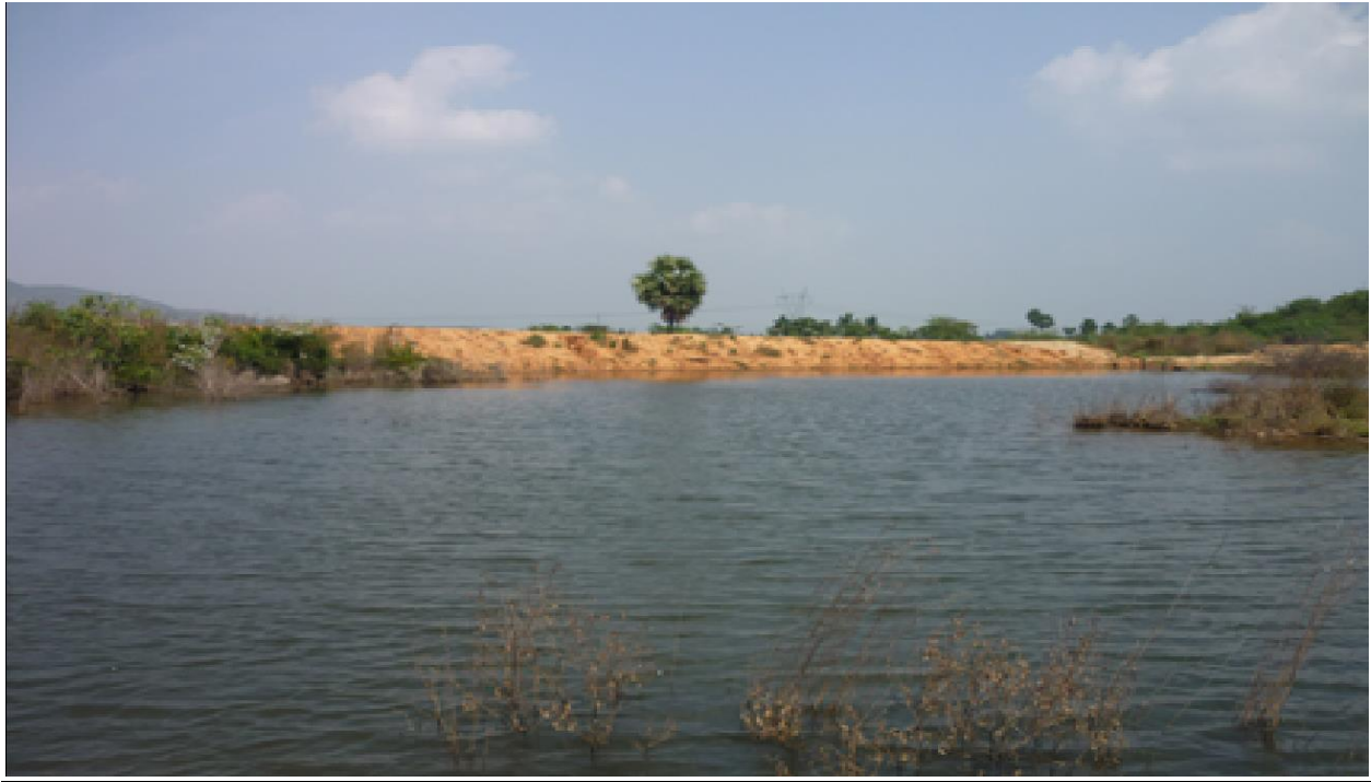
Figure 2: Percolation tank at Pathapelam village in Andhra Pradesh.
